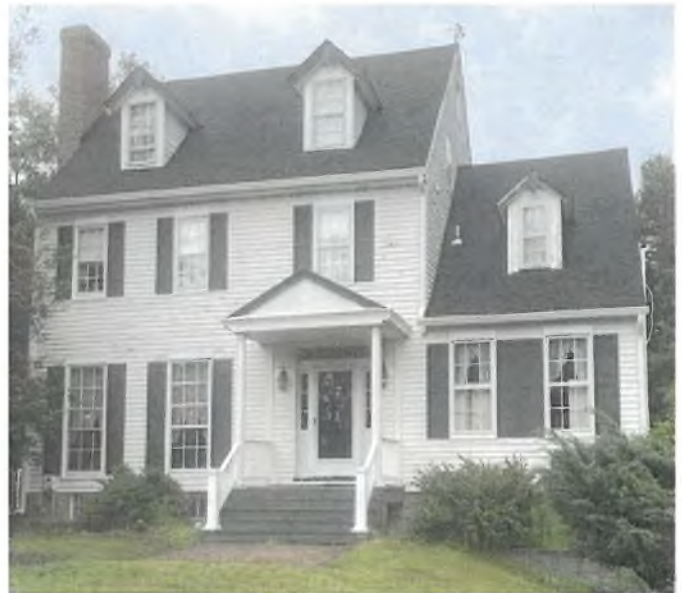
The addition (right) at Calvert Manor, Lower Marlboro is detailed much like the original building. Image courtesy of Calvert County.
