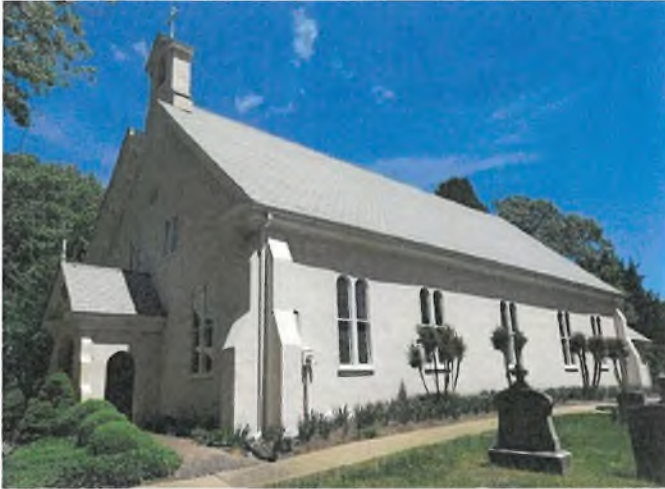
The brick walls of Christ Church, Port Republic were stuccoed over in 1906.
