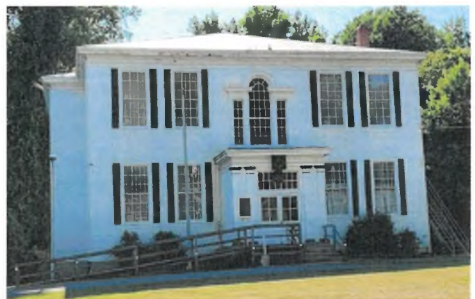
The tall windows are scaled appropriately to the overall size of the Prince Frederick High School building.
