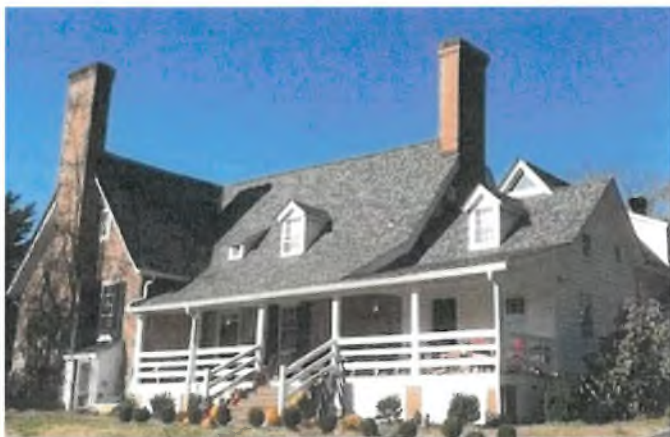
The roof of the main house at Cedar Hill, Prince Frederick has new asphalt shingle roofing to replace the previous asphalt shingle roof. Image courtesy of Calvert County.
