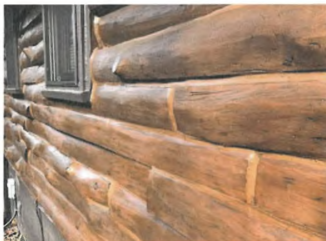
Log repair work at the Schultz Cabin, Port Republic. Image courtesy of Calvert County.
