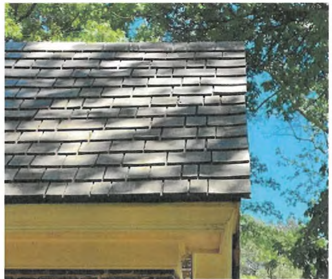
Wood shingle roof of Middleham Chapel, Lusby.
