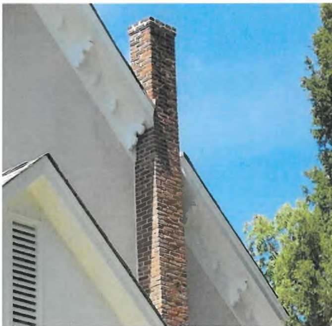
Brick chimney at Christ Episcopal Church, Port Republic.
