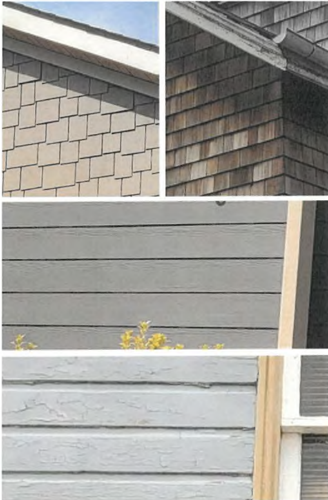
Examples of synthetic materials that are not a good match for traditional materials. Upper left, synthetic shingles are too thin and flat; middle, synthetic siding profile is too narrow and the applied texture does not replicate wood boards well.
