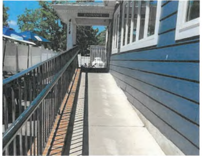
This ADA ramp provides access to the side entrance at this restaurant in North Beach.
