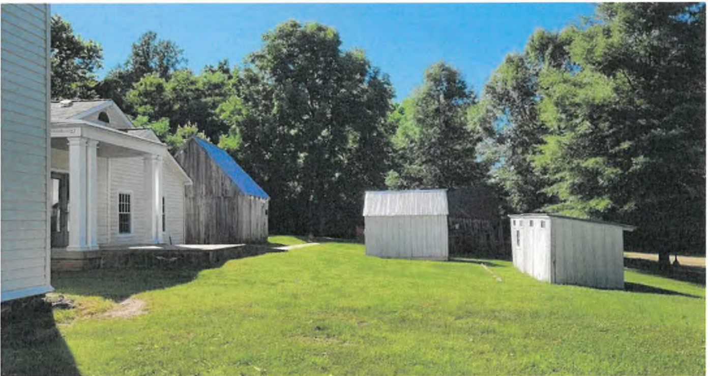
There are ten accessory structures at Linden (also known as the John Gray House), Prince Frederick, including an ice house, smokehouse, servant quarters, corn crib, and poultry house.
