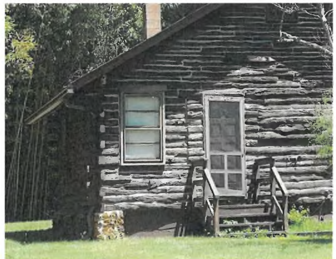
This log home near Port Republic is constructed on stone pier foundations.
