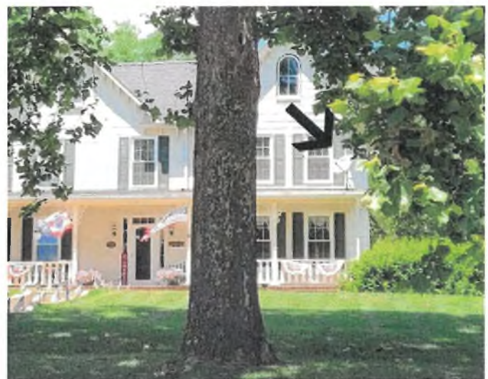
It would be preferable to locate equipment like satellite dishes on a secondary elevation.
