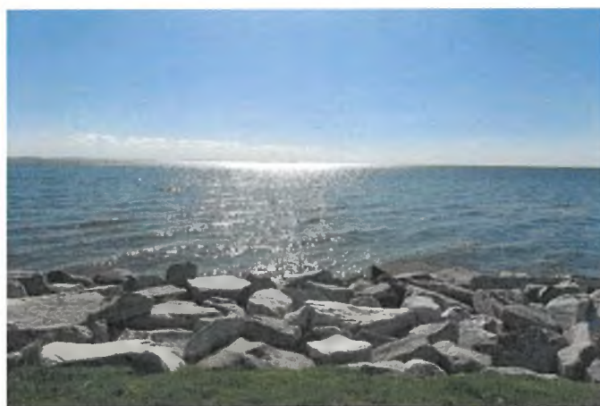
Stone revetment along the shoreline of the Chesapeake Bay at Chesapeake Beach.
