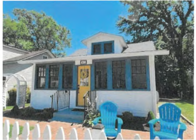
This bungalow on 7th Street, North Beach is clad in aluminum siding.
