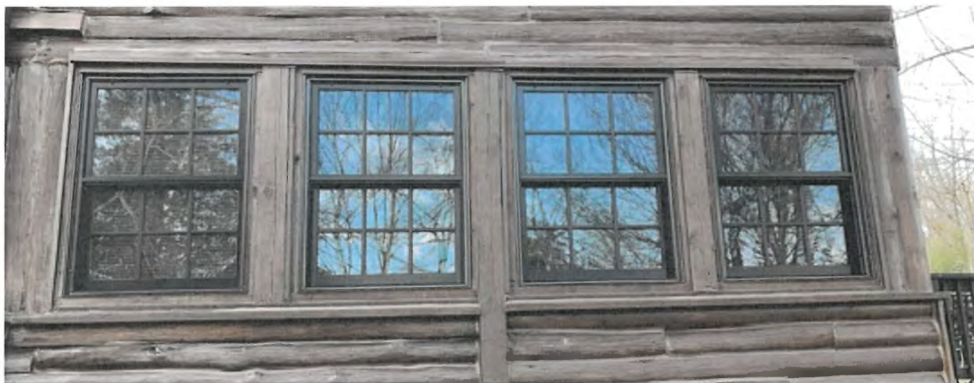
Replacement windows at the Schultz Cabin, Port Republic. Image courtesy of Calvert County.
