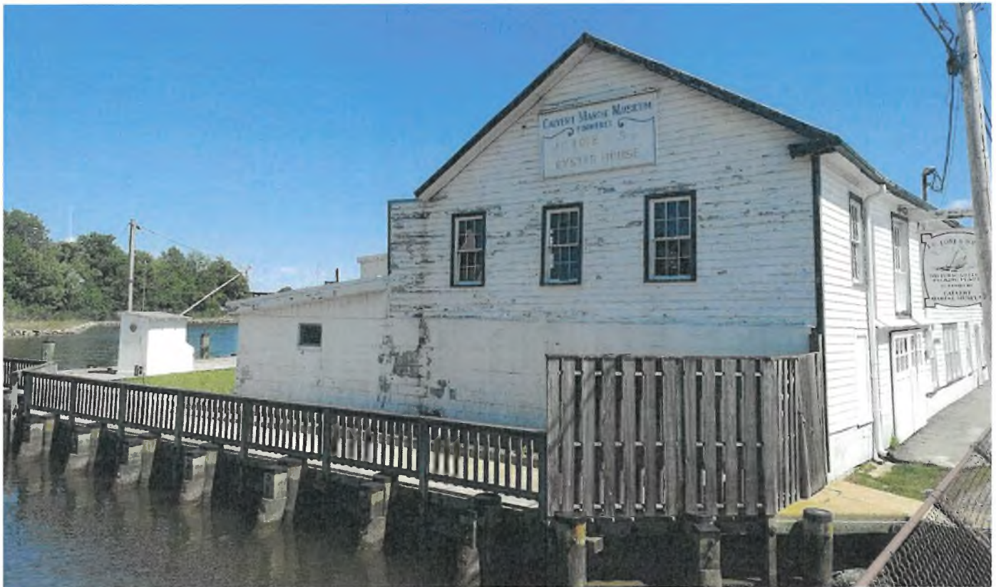
J.C. Lore Oyster House, Solomons sits directly on the Patuxent River and is subject to flooding. The base of the walls up to the bottom of the first-floor windows are constructed of concrete to help withstand the effects of flood water.
