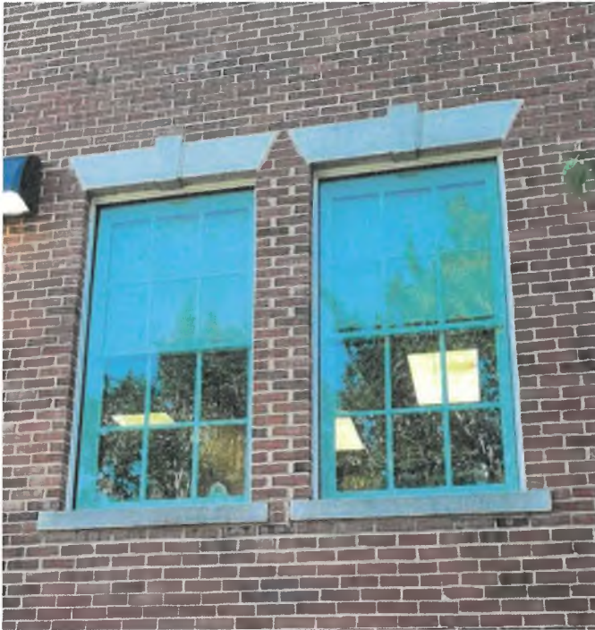
These exterior storm windows do not have any rails to obscure the view of the windows inside.
