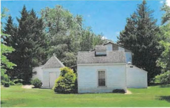
These four accessory structures at the Wilson-Digges House, Owings were constructed after the house was relocated to this site in the 1970s, but they are in keeping with the scale and design of the primary building on the site.
