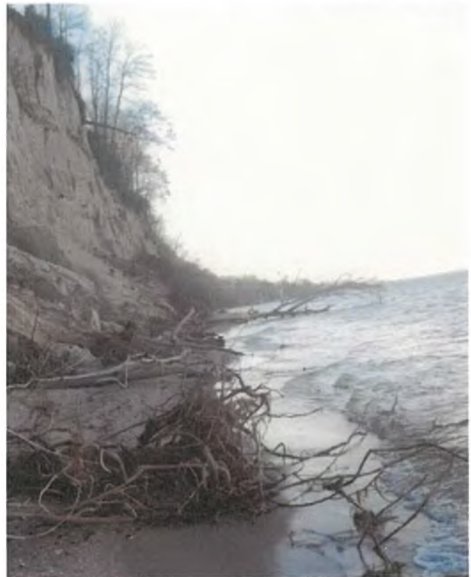
The steep slopes at Calvert Cliffs are subject o severe erosion. Photograph by Bella White.
