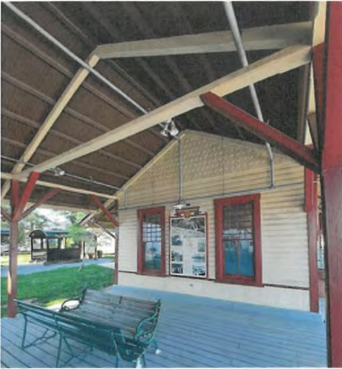
The large roof overhang of the Chesapeake Beach Railway Station, Chesapeake Beach creates a covered gathering space.
