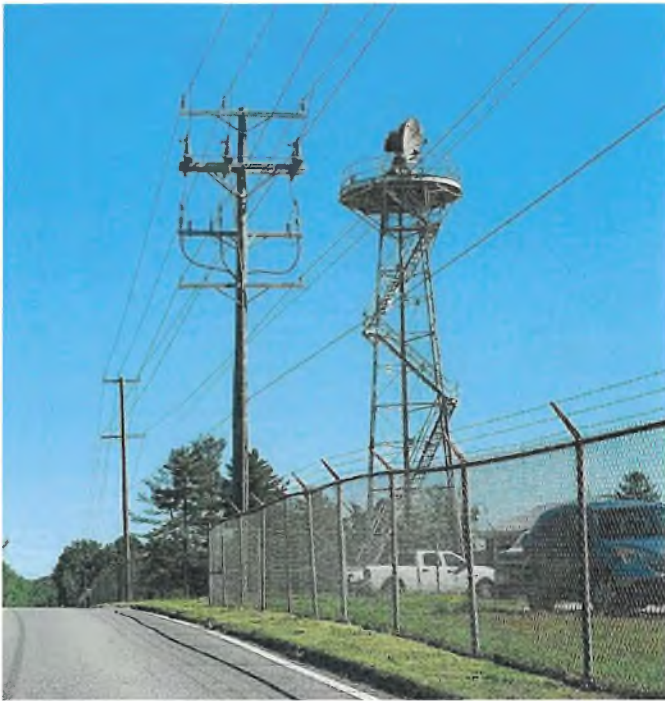
Modern telecommunications and other equipment can be detrimental to historic sites if located with a viewshed.
