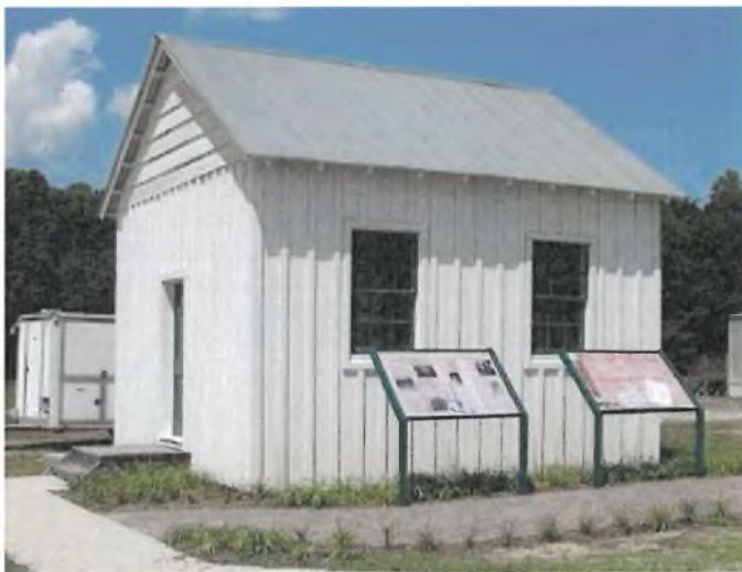
Old Wallville School, Prince Frederick, ca. 1880-1934 is the oldest standing one-room schoolhouse for African American students in Calvert County.
