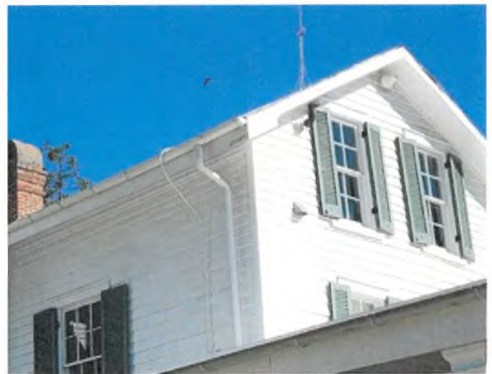
The half-round gutters and smooth round downspouts of Linden (also known as the John Gray House), Prince Frederick are in keeping with the character of the Historic District.
