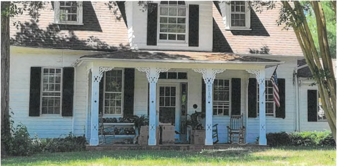
Distinctive front porch detailing on the Mills House, Lower Marlboro.
